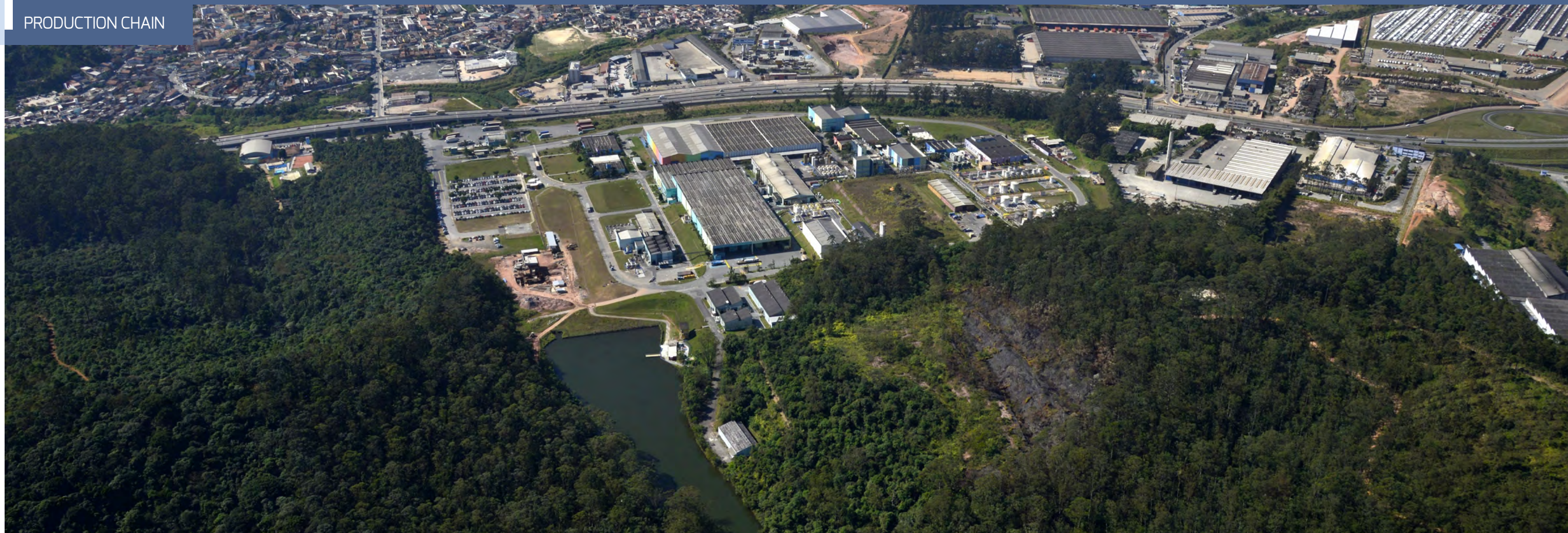
AERIAL VIEW OF THE AKZONOBEL FACTORY NEXT TO THE RESERVATION
